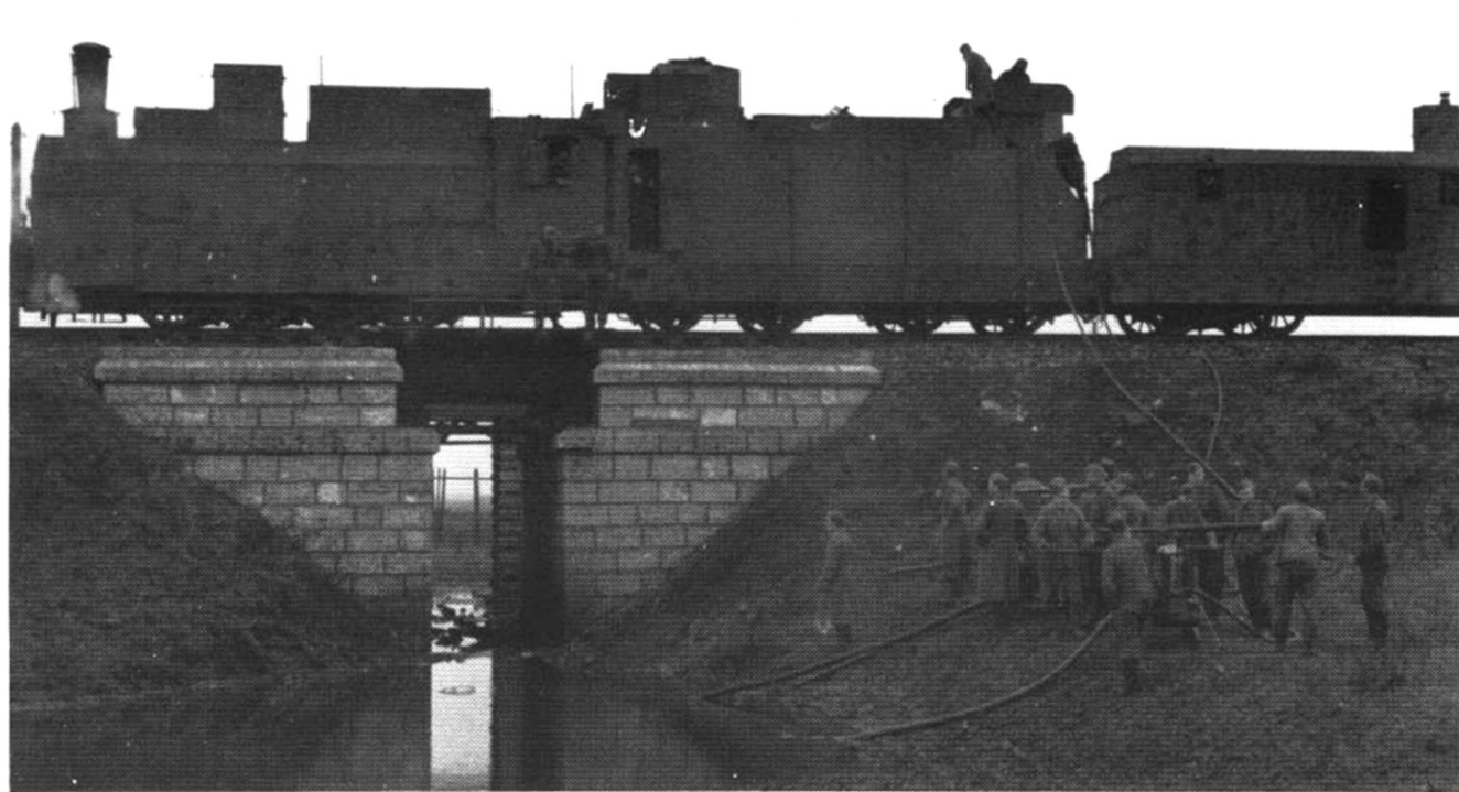
This is why the water tanks often had to be filled from bodies of water underway, using pumps brought along for that purpose. The pictures above and below show such an emergency supplying of Armored Train No. 28. (BA)
