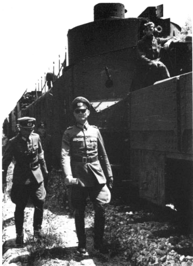
Left: the rear part of Armored Train No. 22, which is being inspected by a commanding general: this artillery car carries only one 7.5-cm gun (note the machine-gun port); in front of it is the command car with the antenna running around the roof. (BA)
